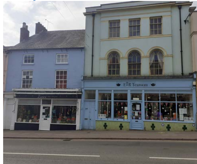
Traditional Treatment to Ground Floor Unit on High Street
