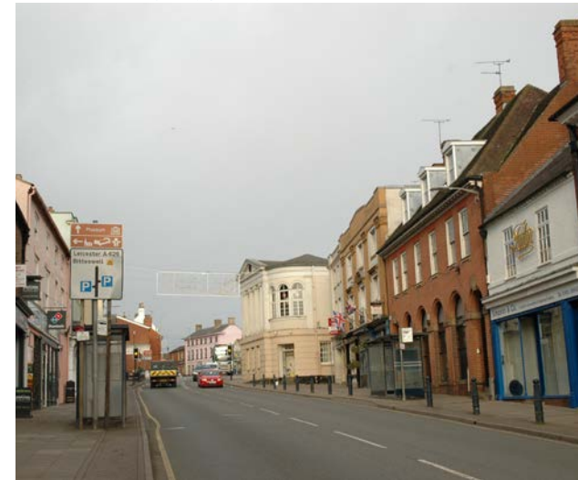
High Street, view north
