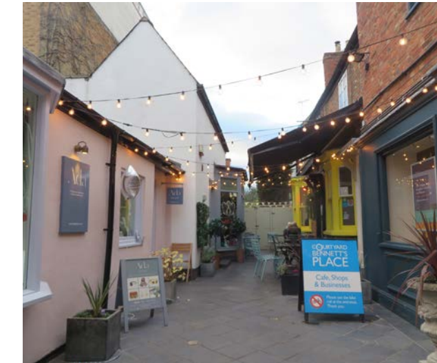
Canopy to shopfront in Bennett's Place, High Street, Market Harborough
