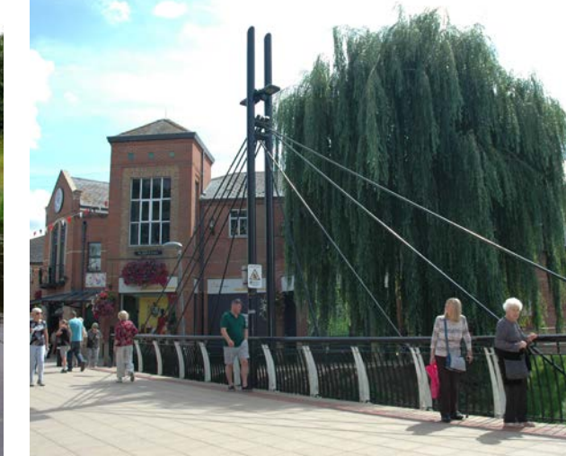
Pedestrian bridge over the River Welland
