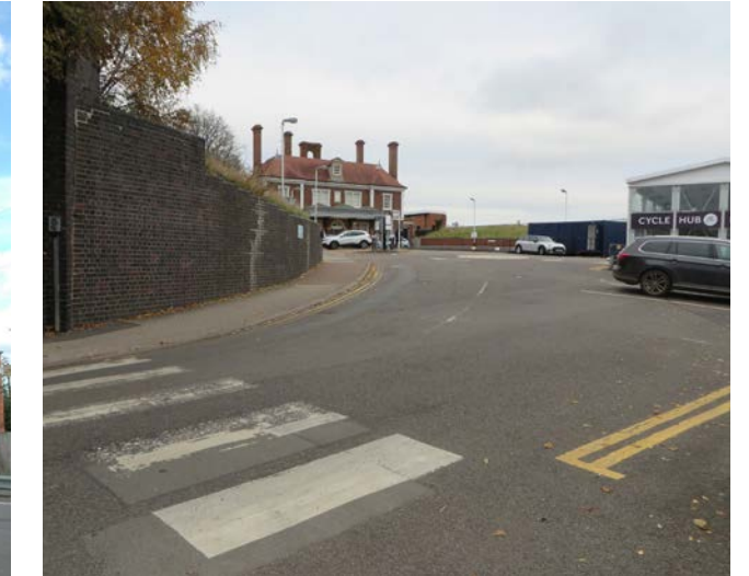
Railway station approach
