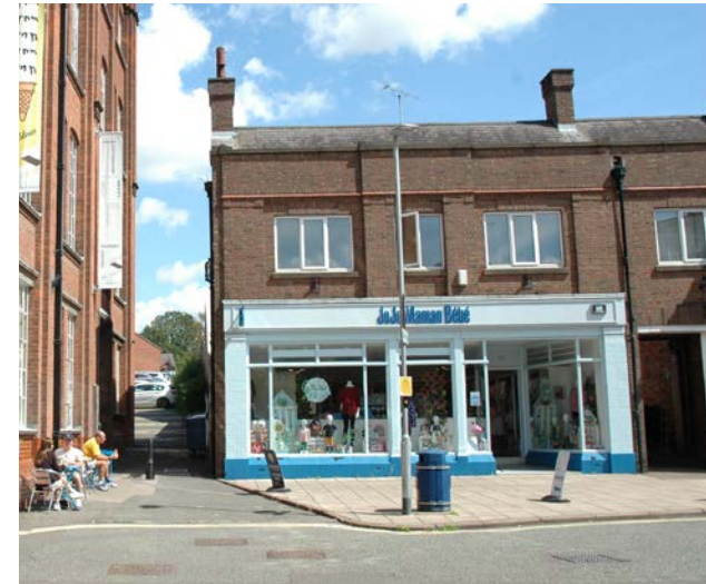
Example of well-articulated window details and recessed doors on Adam and Eve Street
