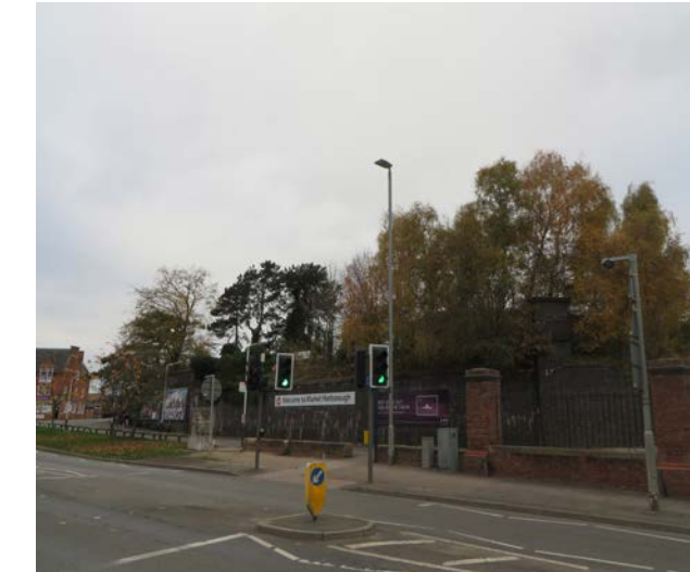
Opportunity to refurbish retaining wall and manage vegetation above
