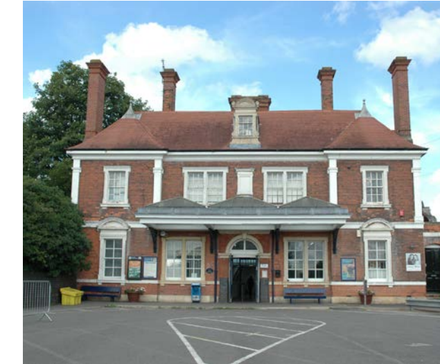
Railway station elevation
