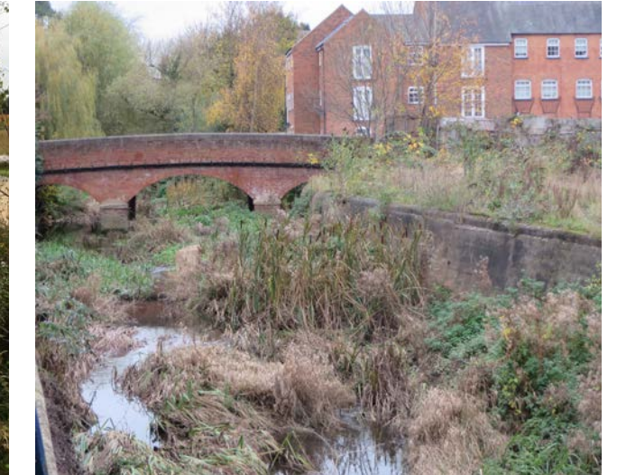
Welland east of Kettering Road bridge
