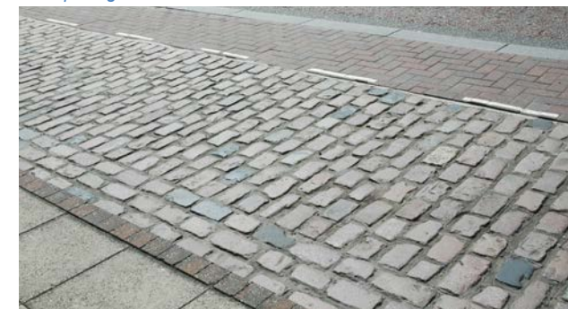
Street parking bays – mix of natural stone and concrete based materials
